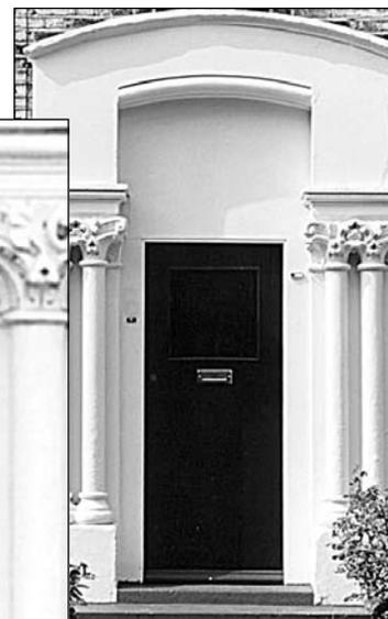
*Centre: An example of the original style of door used on the estate. This one is of the four panelled half-glazed variety. Cheaper modern four panelled doors often with sloping upper panels do not recreate the moulded, heavy character of originals and so are not acceptable.*
