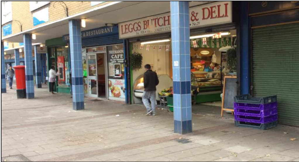
11-33 Freemasons Road (LBN photo)
