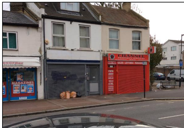
93-95 Vicarage Lane (LBN photo)
