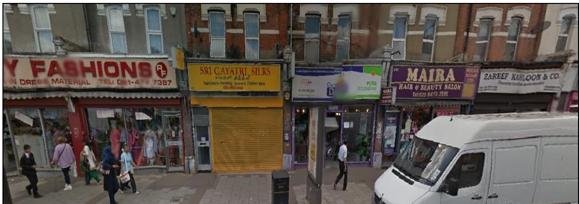
328-348 High Street North (Google)
