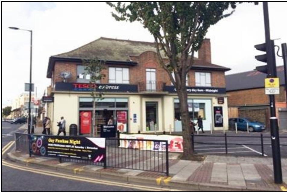
Former Pub (Tesco's) 523 Greengate Street (LBN photo)
