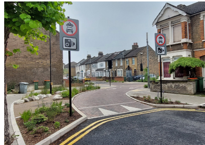
Keogh Road modal filter, implemented as part of Atherton LTN following decision to make the LTN permanent
