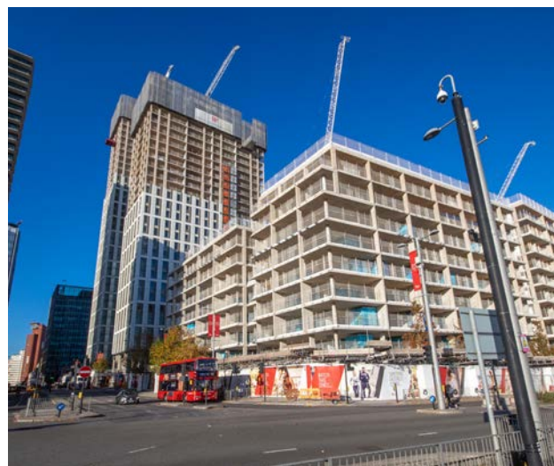
Image: Cherry Park progress on site (December 2021)
