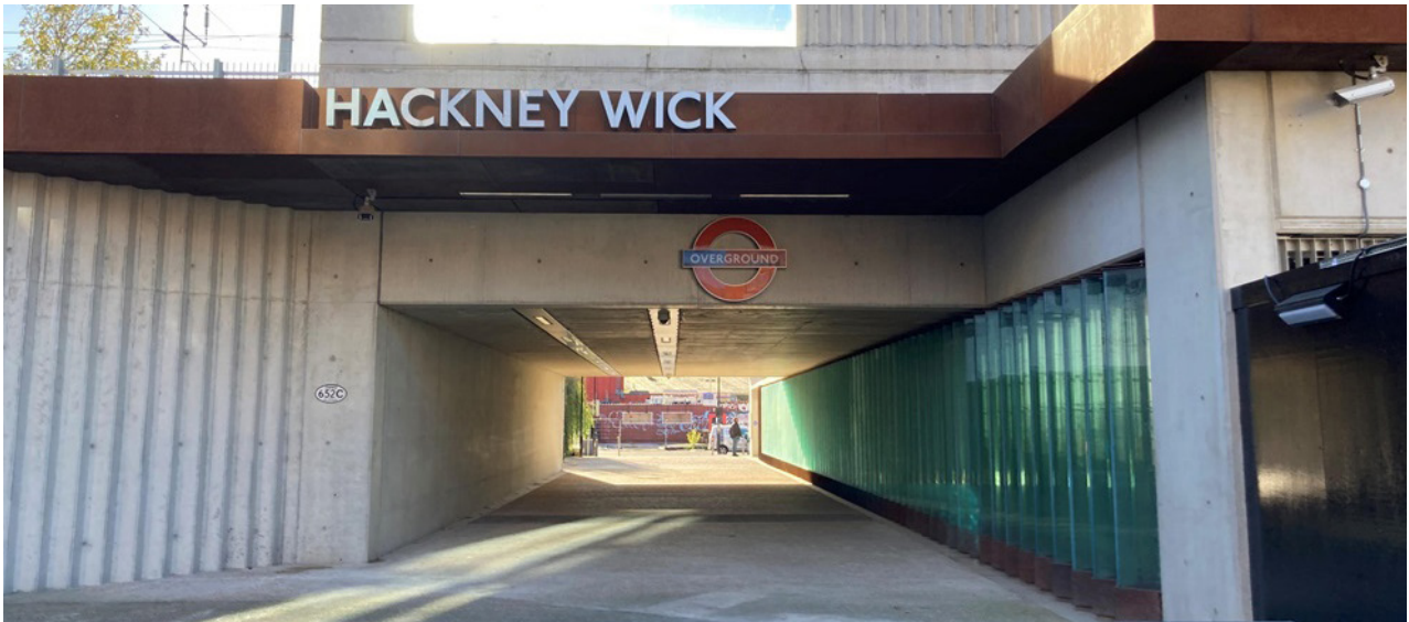
Image: The new route created through the improvements to the Hackney Wick station
