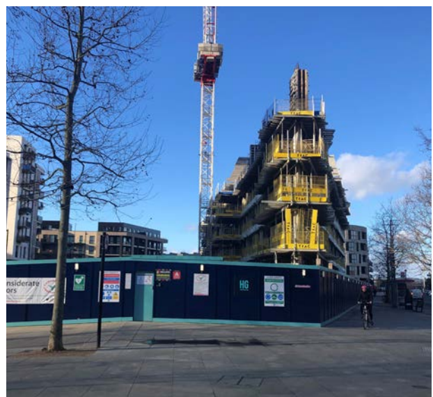
Image: East Village N05 progress
