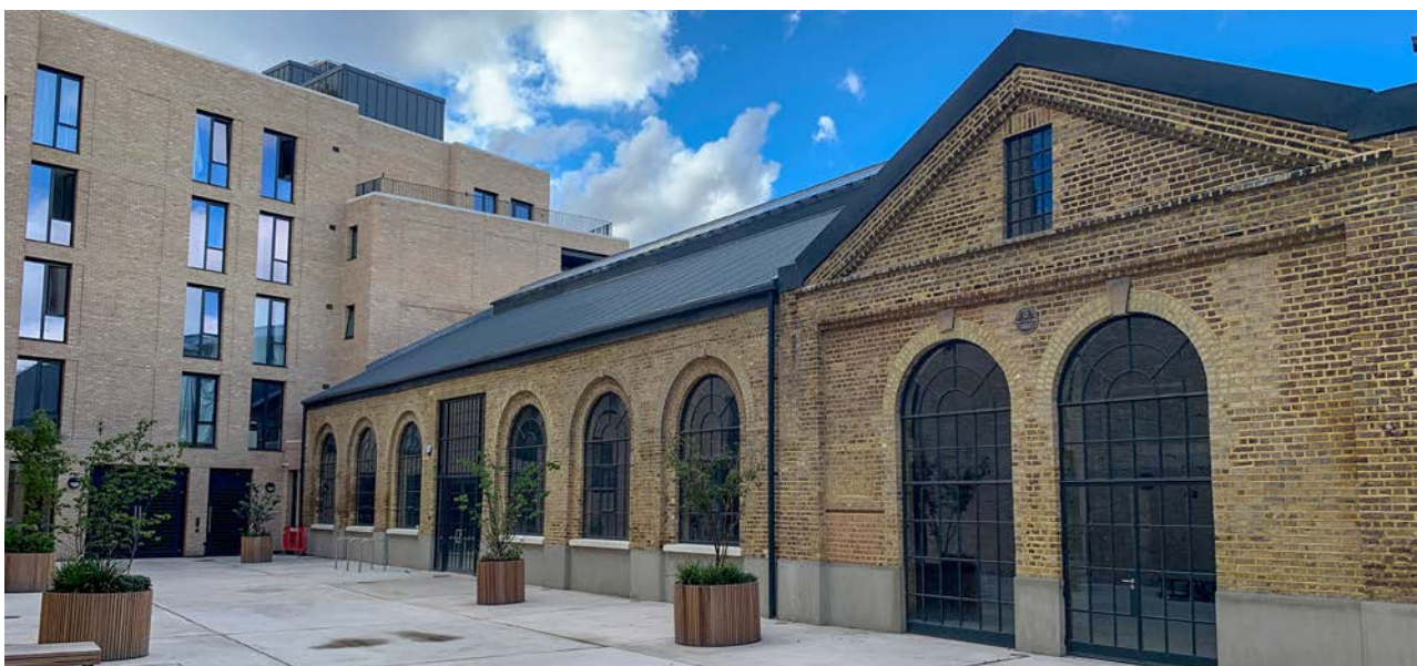
Image:57 Berkshire Road (ref: 16/00704/FUL), employment floorspace. Delivered in 2020/21
