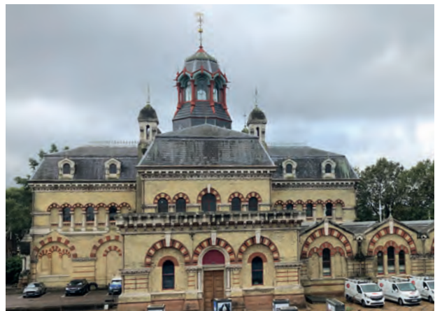
Above: Abbey Mills Pumping Station
