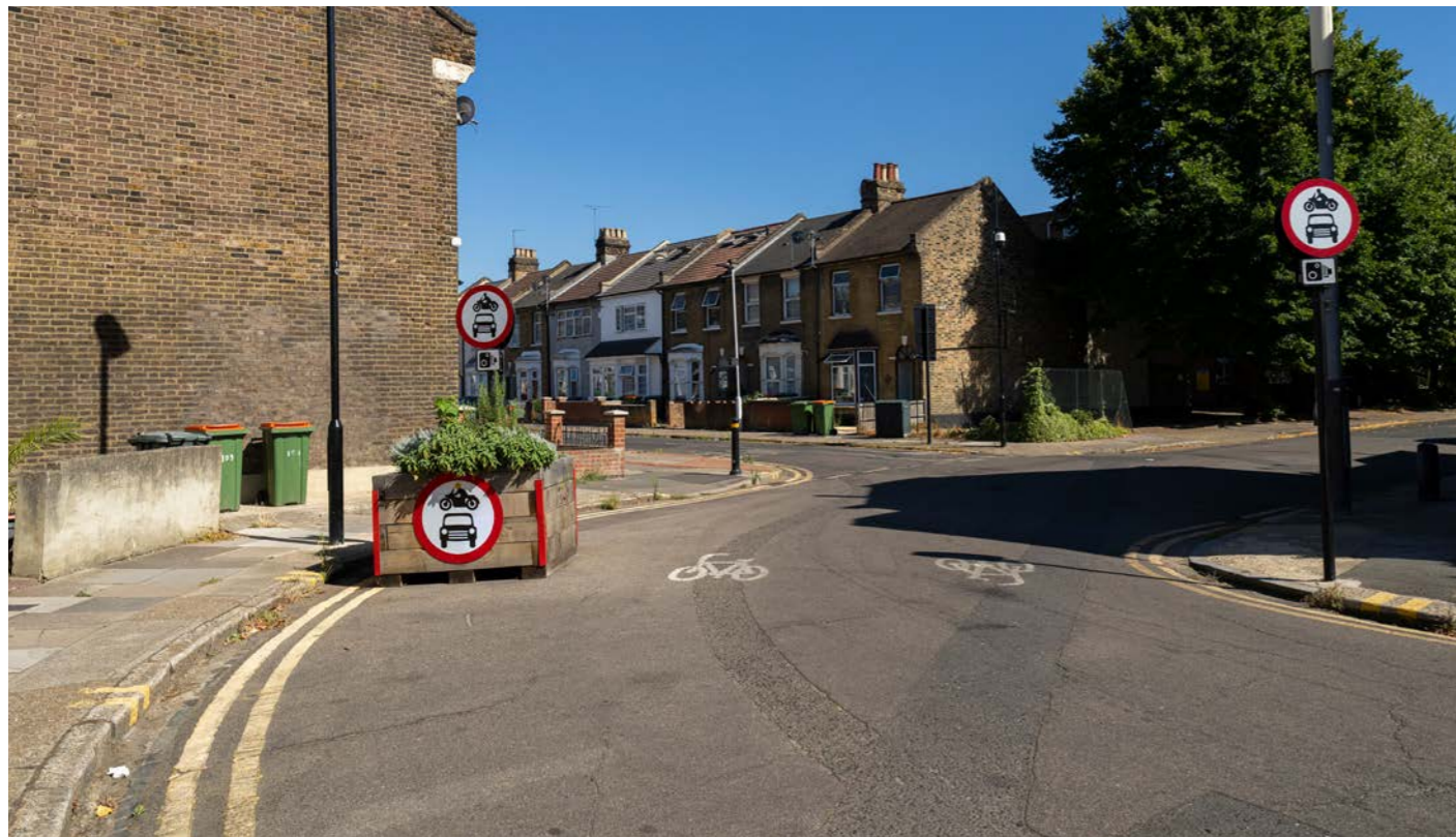
Keogh Road modal filter, implemented as part of Atherton LTN during experimental stage
