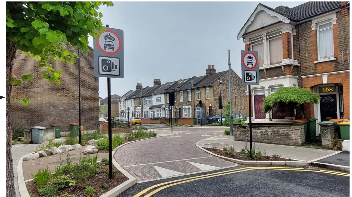
Keogh Road modal filter, implemented as part of Atherton LTN following decision to make the LTN permanent
