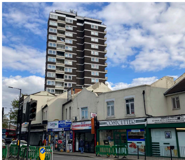
Fig 19 Isolated tall building impacting Plaistow High Street character
