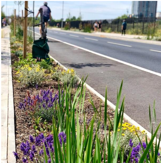
Figure 70: Rain gardens installed in Waltham Forest (Source: Meristem Design)
