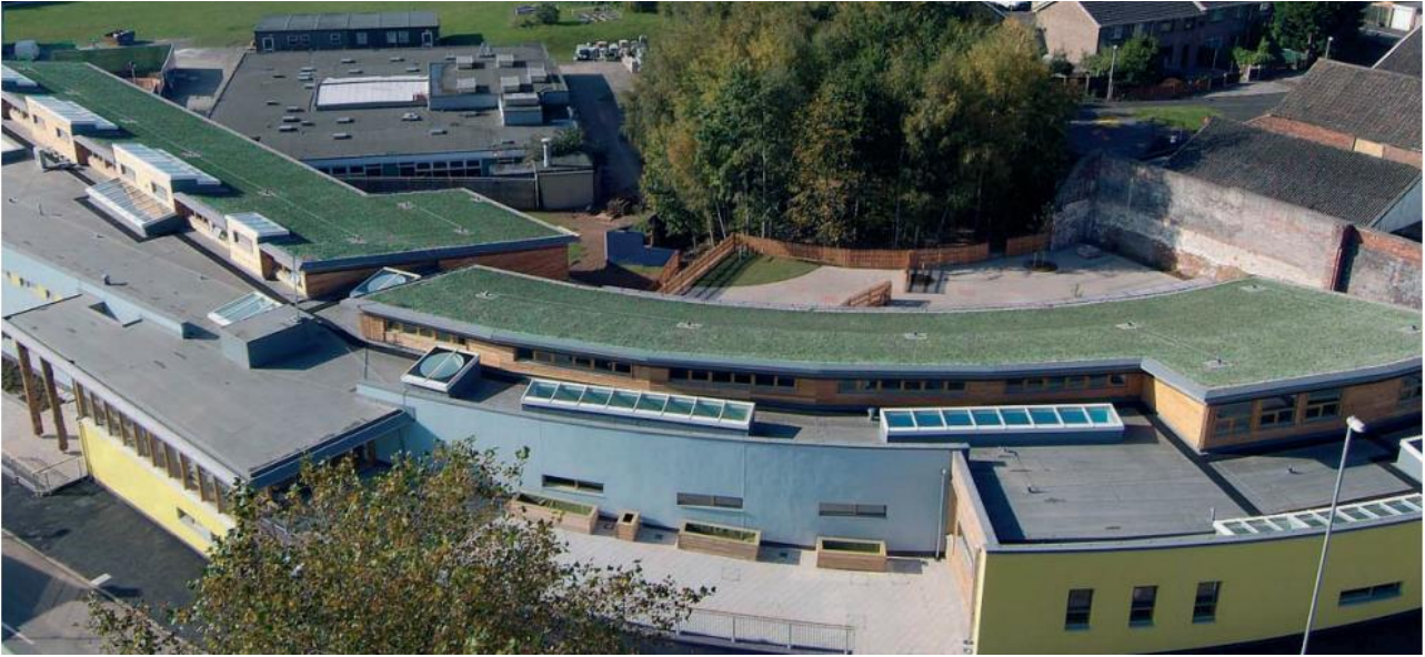
Figure 75: Example of a green roof (Source: Bristol Council SuDS Case Studies https://www.bristol.gov.uk/files/documents/2709-woe-suds-case-study-04-barton-hill-green-roof/file ).
