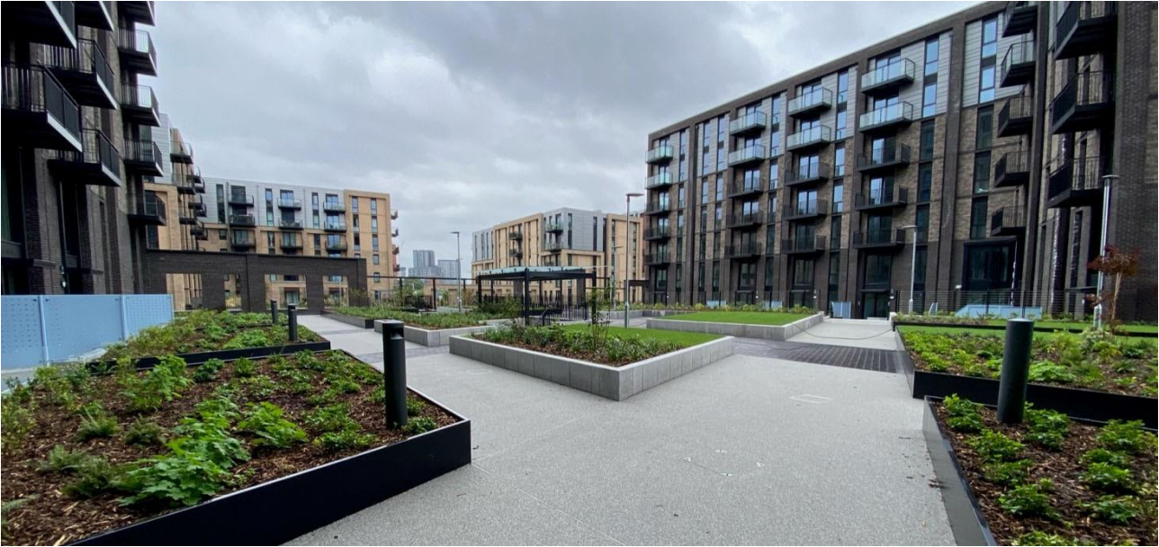
Figure 71: Podium deck blue roof in dense urban development, Middlesdick, Salford (image: abg geosynthetics).
