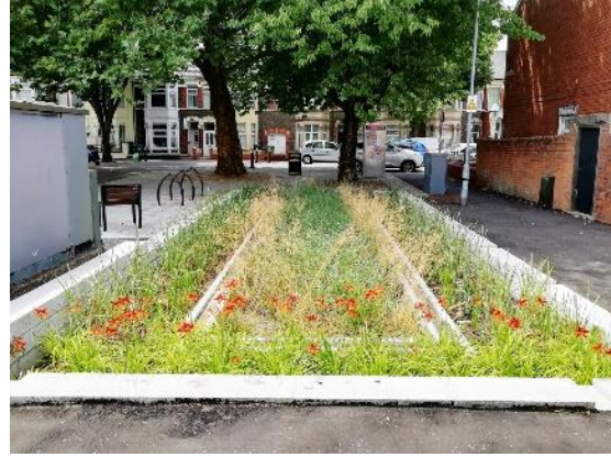
Figure 77: Example of an infiltration basin (Source: Arup).
