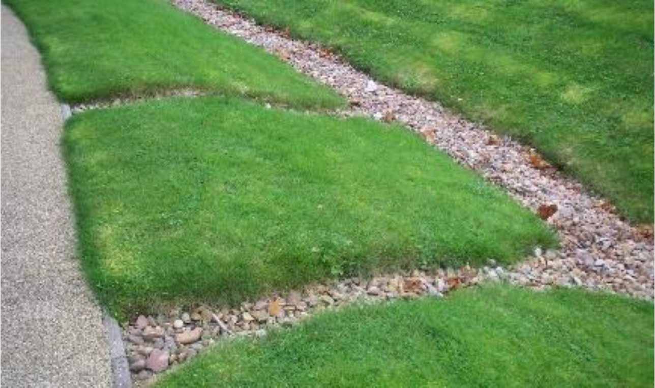
Figure 74: Example of a filter drain (Source: Arup).
