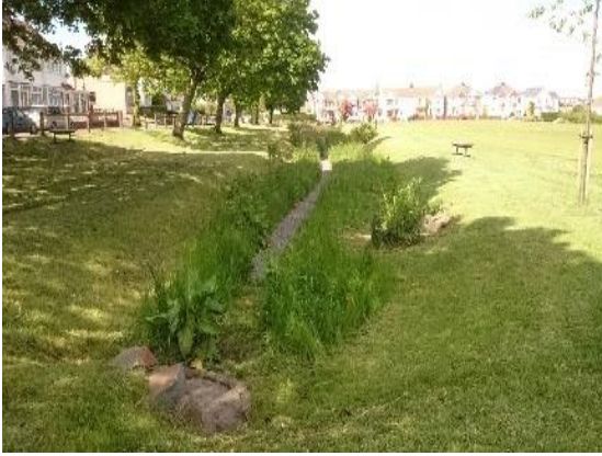
Figure 76: Example of soakaway (Source: Arup).
