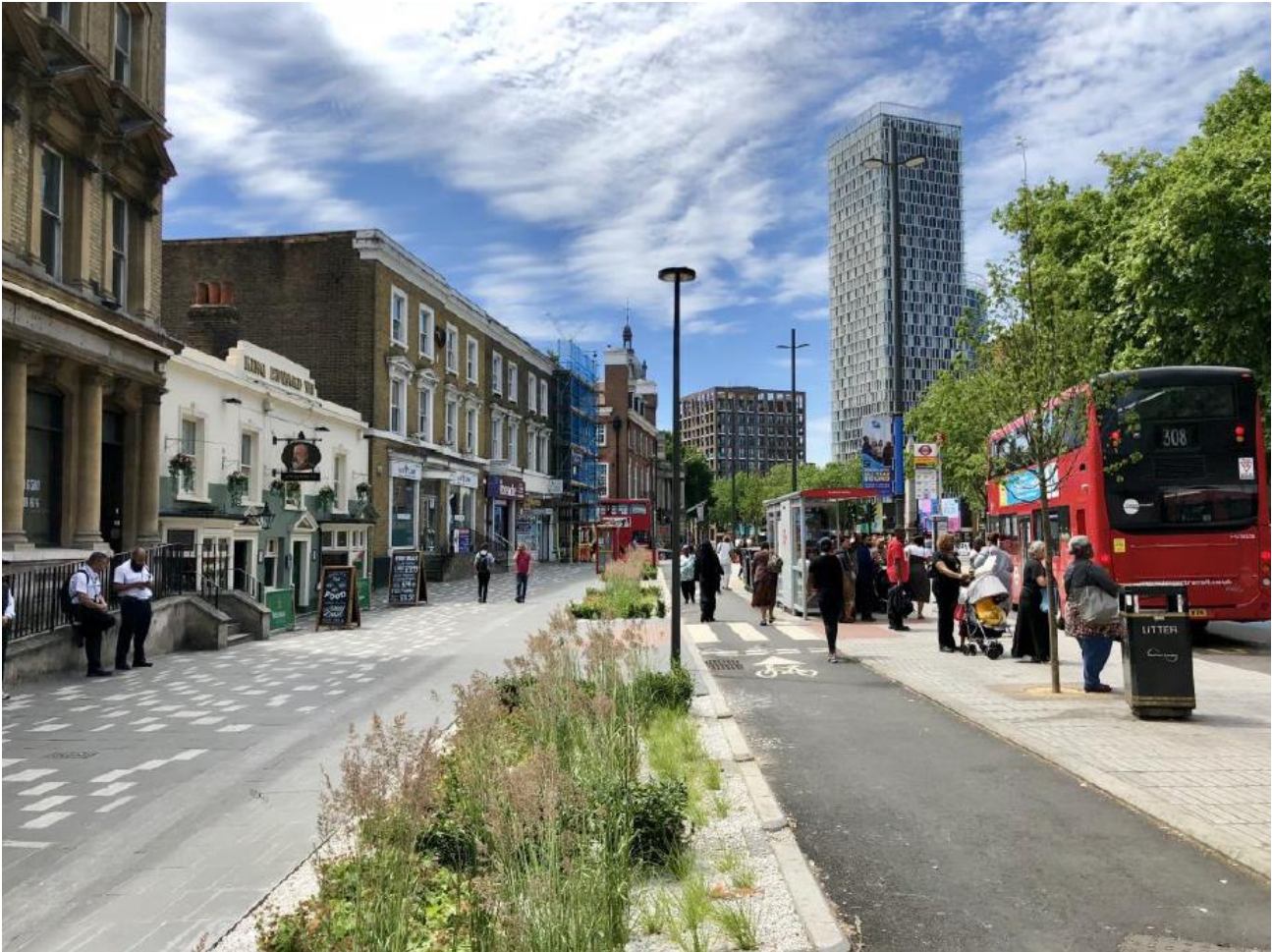
Figure 8-1: Rain garden planted as part of the Stratford Gyratory SuDS project (2018) (Source: London Borough of Newham Council).
