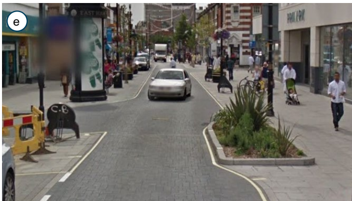
Extend existing SuDS treatments
