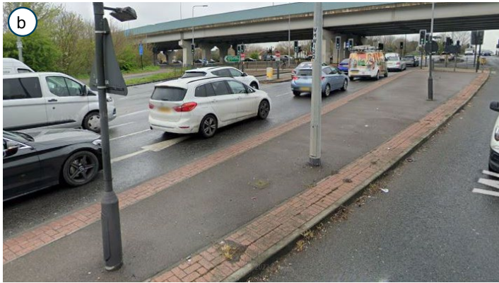
Install ground plane planting to improve aesthetics
