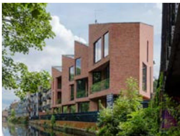
Old Ford Road - pH+ Architects
