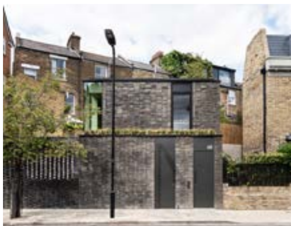
Sandbrook House - Ellis Miller and Patners
