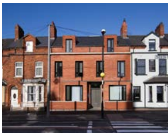
Home for Home RVH - McGonigle McGrath Architects
