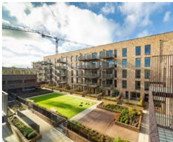
Beckton Parkside orients private amenity spaces and more sensitive internal residential uses away from the A13. Beckton, Newham.
