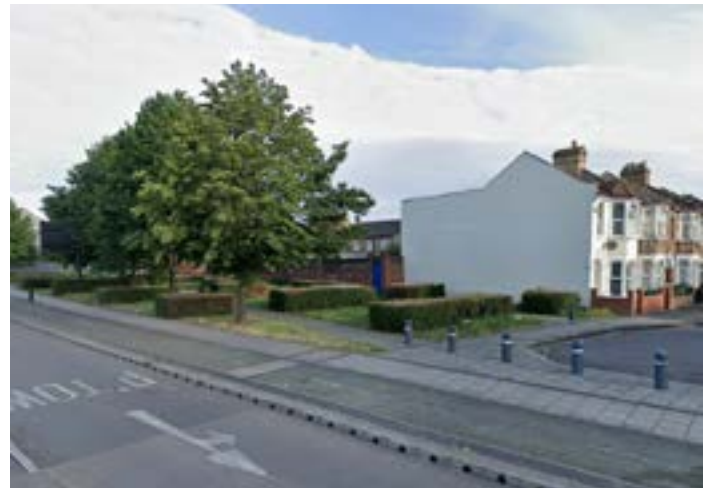
Developments along A13 incorporate a green buffer to protect surrounding homes, gardens and streets from poor air quality.
