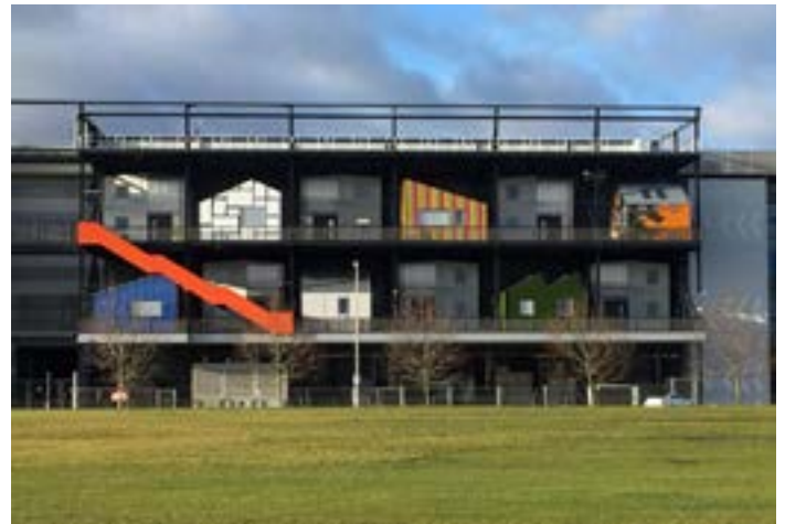
The Gantry animated façades provide visually attractive frontage for creative studios, Here East Hackney
