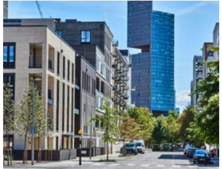
The emerging Chobham Manor neighbourhood provides a mix of tenures and typologies that delivers medium to high-density development alongside quality public realm and communal amenity spaces.
