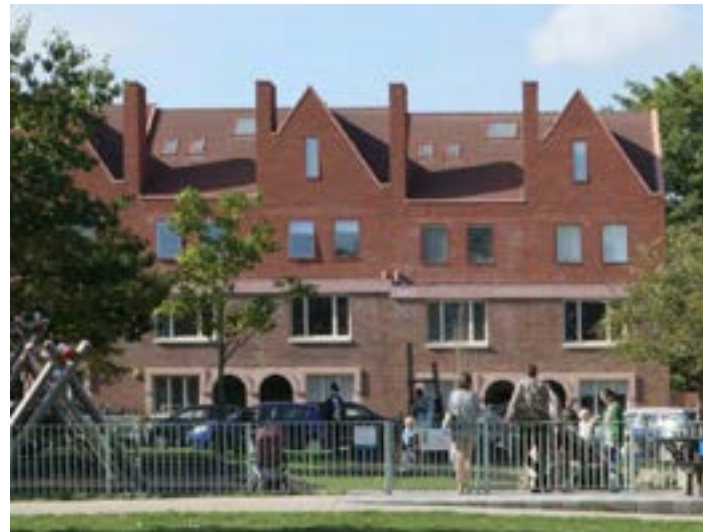
This contemporary arts and crafts style apartment block successfully accommodates its upper levels within the roof form in an area characterised by two and three storey terraces. The material choices, simple detailing and projecting gables reduce the impact of the increased scale and massing. Nunhead Green, Peckham by AOC architects. Photo credit: David Grandorge.
