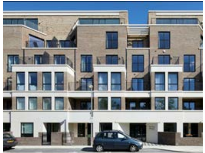
The massing strategy and facade design for Park View Mansions, Chobham Manor accommodates 6 storeys in a way that reduces visual bulk and carves out areas of private amenity use; an asset especially important for high density living. Photo credit: Haworth Tompkins.
