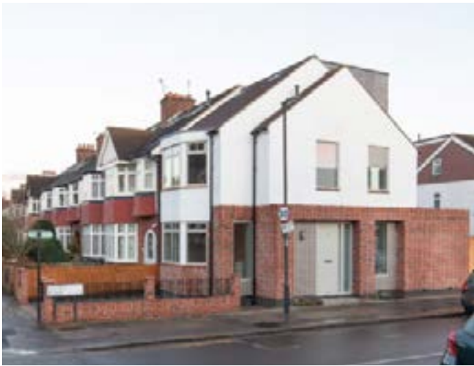
A new dwelling house delivered on a narrow end of terrace site. A bay window and fenestration continue the rhythm of the primary street frontage, whilst access to the dwelling is on the gable end. Massing and building line is stepped back to create subservience, whilst the material palette complements the existing terraces. Lucien Road, Wimbledon Park by Harp and Harp architects. Photo credit: Adam Scott
