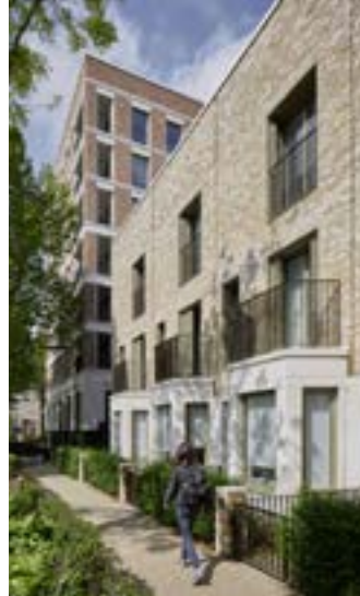
A terraced house with projecting bay window, first floor balcony and soft landscape boundary and defensible zone.
