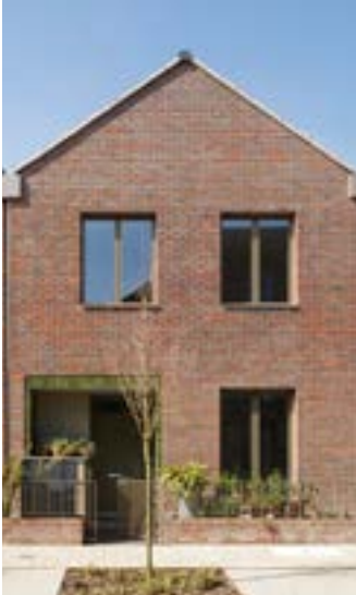
A terraced house with recessed porch, integrated storage, large ground floor window with deep reveals; and hard landscape boundary and defensible zone.
