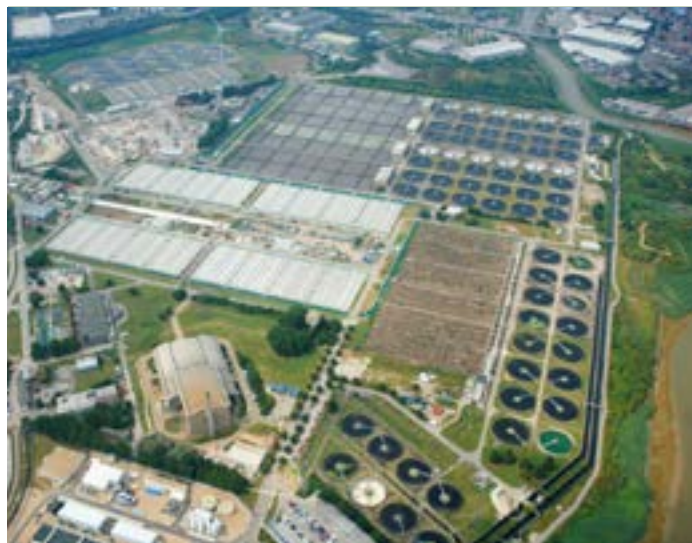
Beckton sewerage treatment plant
