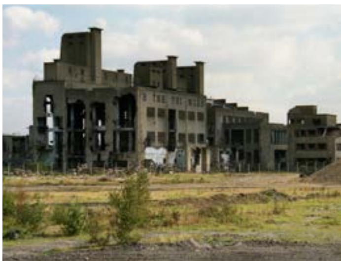
Former Beckton gas works.
