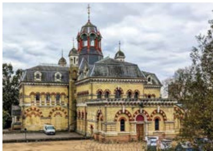
Abbey Mills pump station
