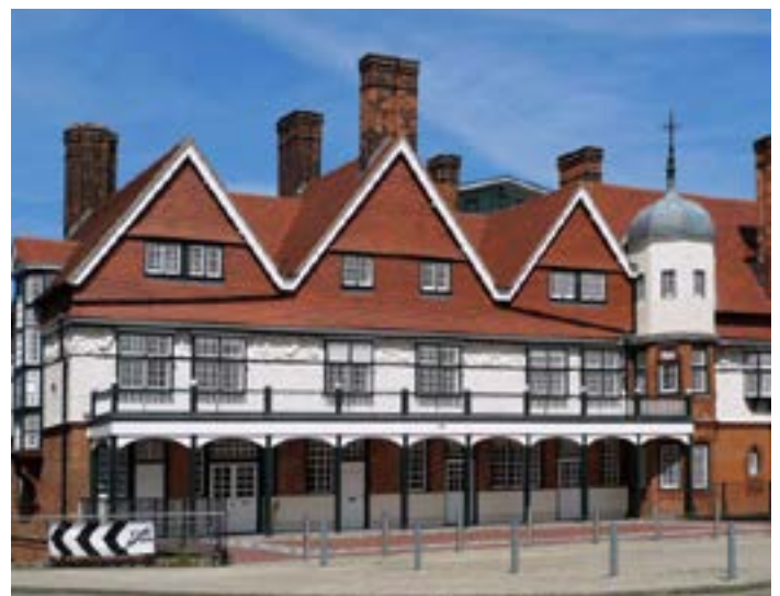
Grade II listed Gallions Hotel was built between 1881 and 1883.
