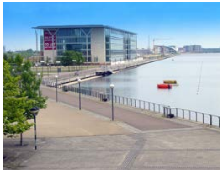
London Borough of Newham offices facing Gallions Point Marina
