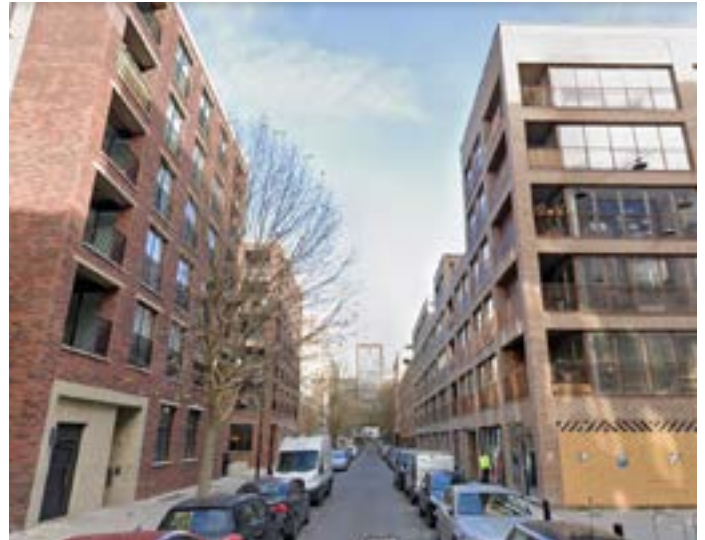
Contemporary and mid-rise residential apartments
