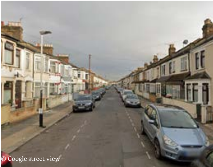
© Google street view Typical historic terraced housing - Whyville Street
