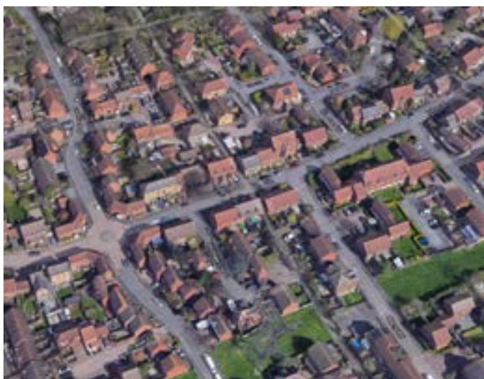
Curved street grid with post war estate housing.
