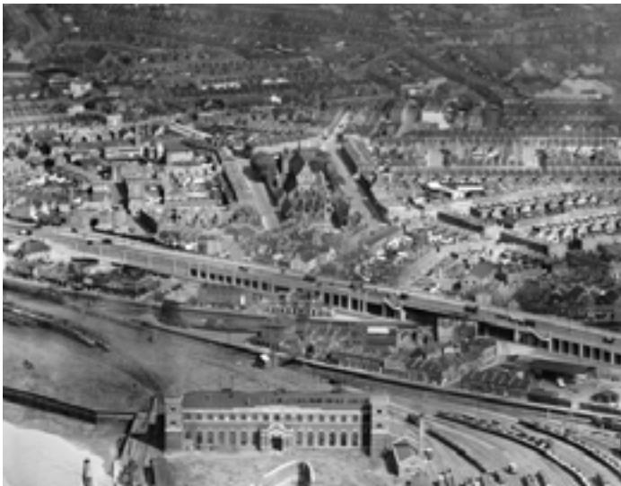
Silvertown Way viaduct
