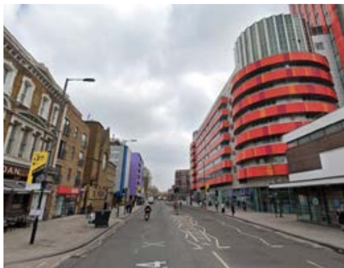
Barking Road with ground floor retail.
