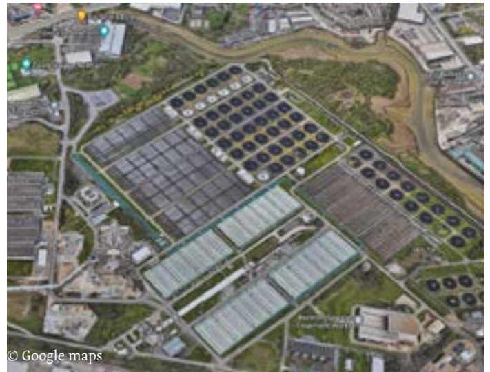
Beckton Sewerage Treatment Works.
