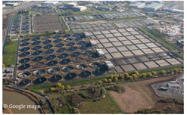
© Google maps Beckton sewage treatment works and desalination plant
