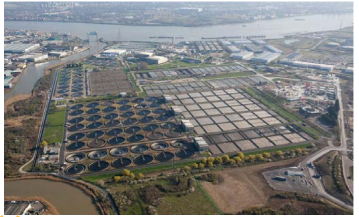
2 Beckton sewage treatment works and desalination plant
