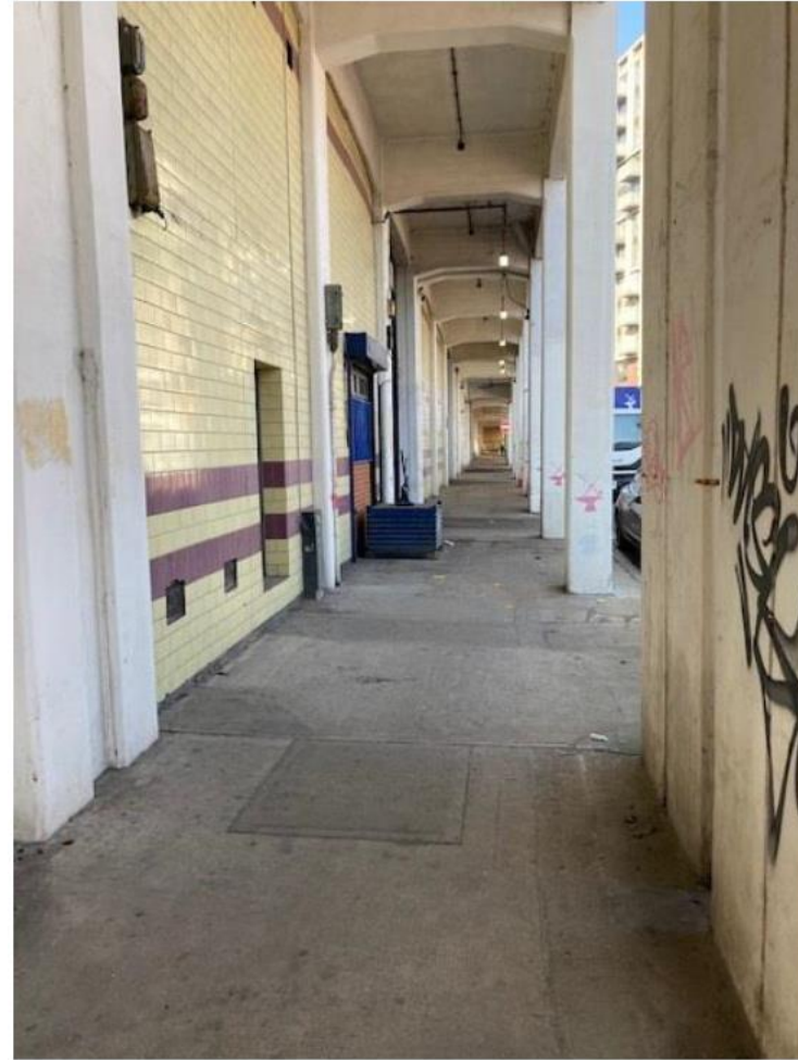
Figure 10: Silvertown Way arches looking North West
