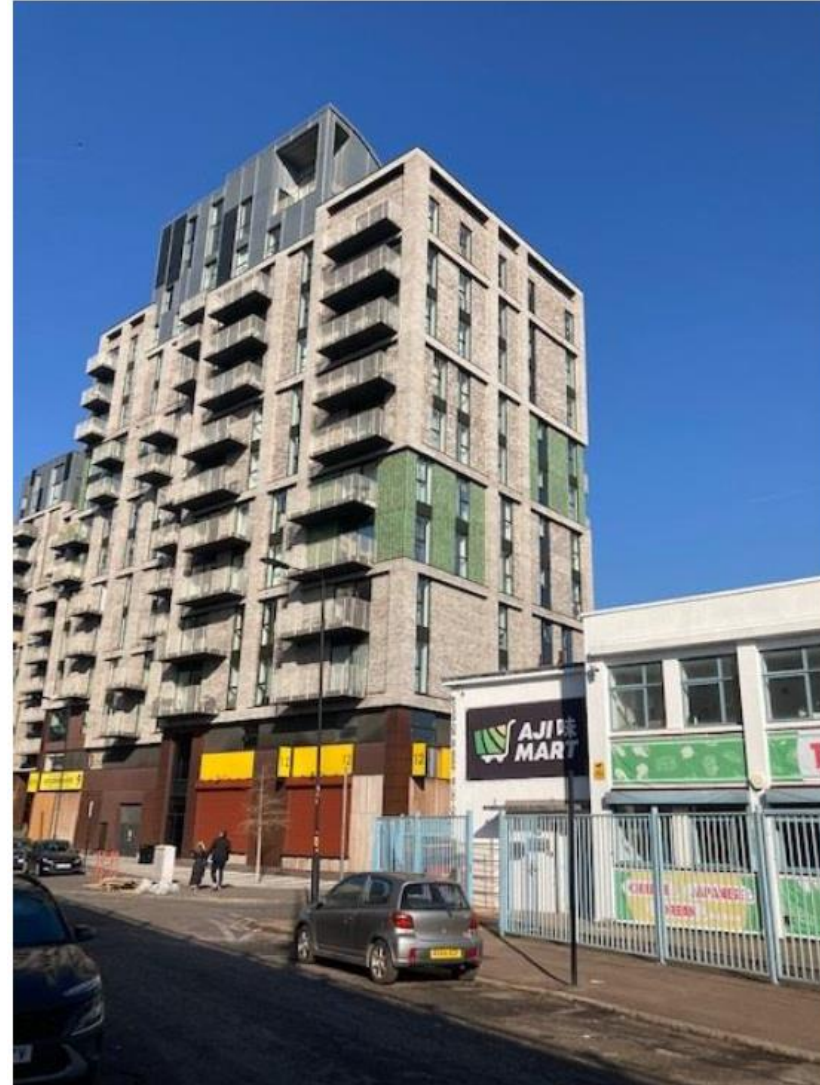
Figure 9: View towards intersection of Caxton Street North and Nelson Street
