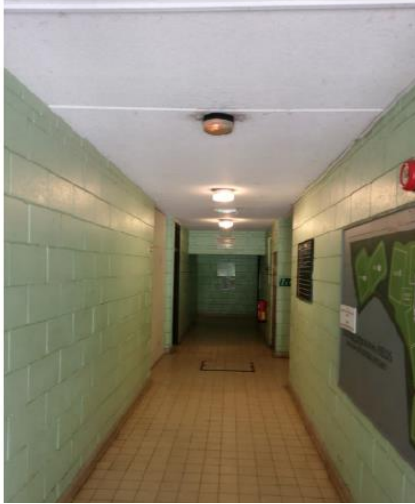
Existing Typical Corridor
