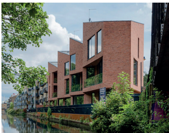
This awkward infill site between a canal and road exploits the constrained geometry, using this to shape the unique, angular footprint, massing and roof form.
