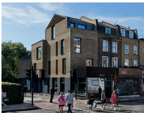
This end of terrace infill includes commercial use at ground floor to continue the high street frontage, with residential on upper levels. The full depth of the plot is utilised by stepping massing back and down.
