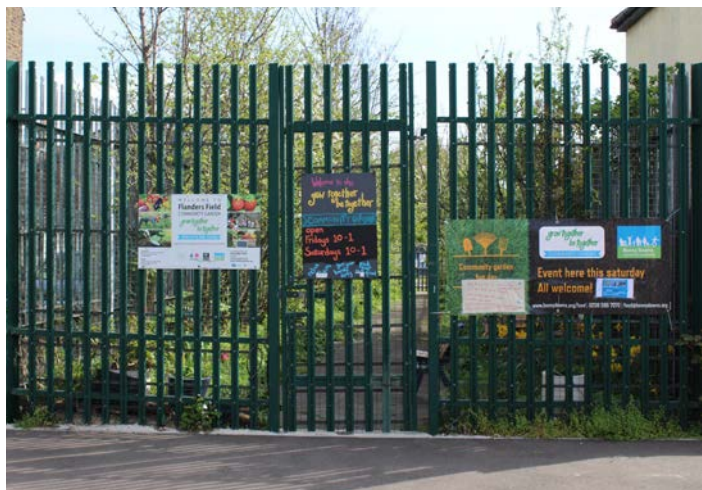
Gate East Elevation
