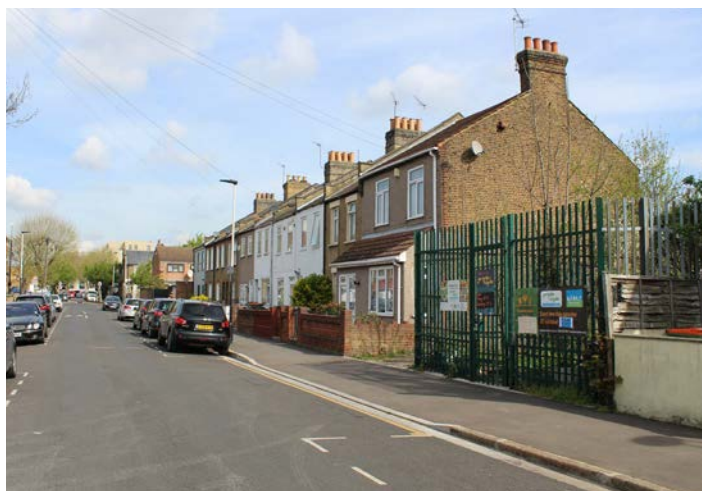
Street view from Wellington Road
