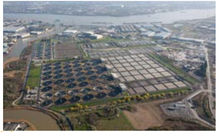
2 Beckton sewage treatment works and desalination plant
