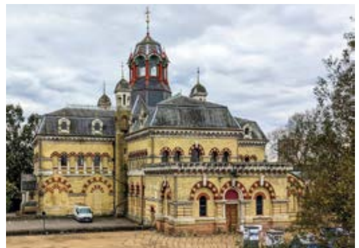
Abbey Mills pump station
