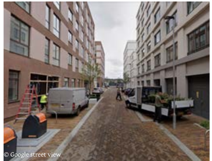
New residential development at Carpet Street on land was previously industrial.
