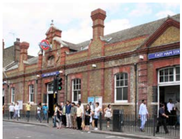
East Ham station and high street
