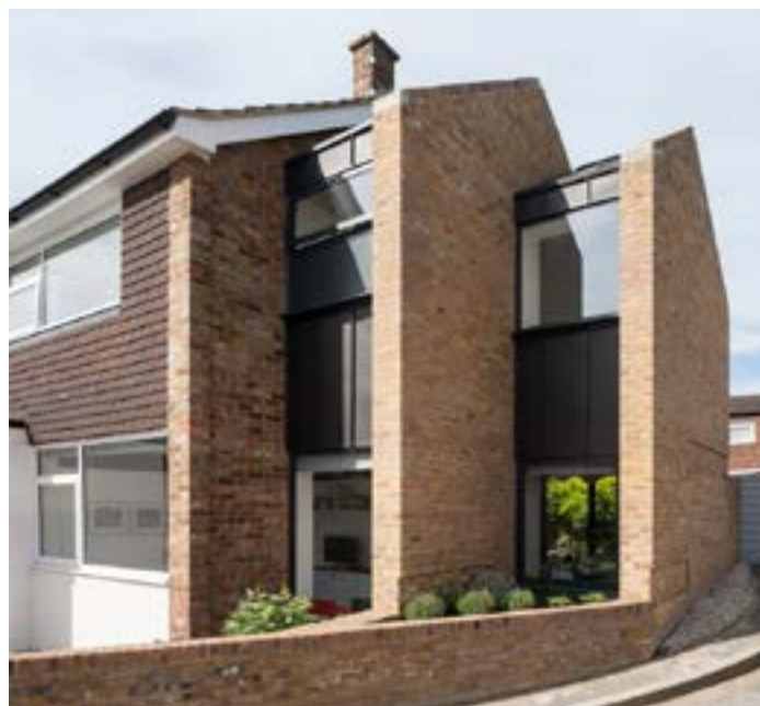
Side extension to a semi-detached dwelling that successfully adopts the principle of subservience by stepping back the front building line and scale, as well as introducing increased volumes of glazing to reduce the visual bulk of the addition. A contemporary material choice also successfully complements the tone of the original building. Wolfram Close, Lewisham by Selencky Parsons. Photo credit: Andy Matthews .
