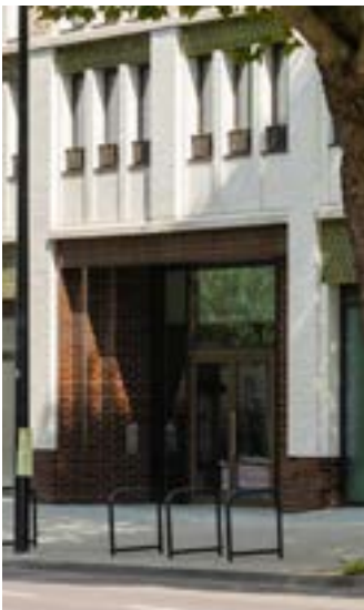
A well lit and semi-recessed communal entrance to high density apartment block, with no defensible zone needed.
