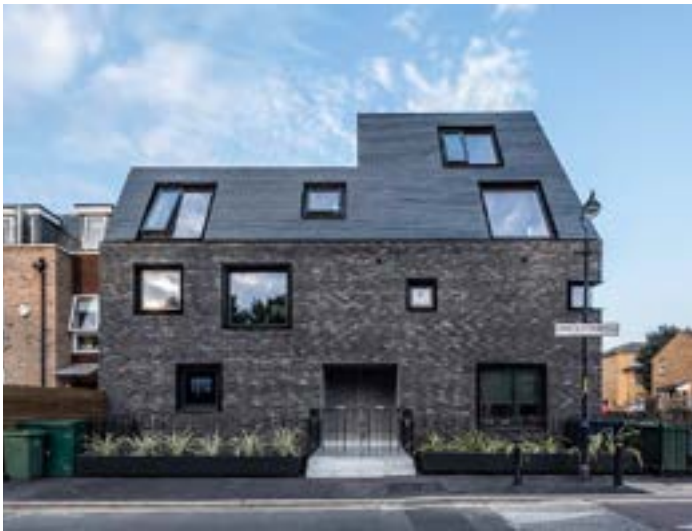
This corner site steps up scale improve local legibility within a low scale context. The mass is broken down by stepping down to the scale of neighbouring properties. Upper levels are successfully contained within the roof form to reduce the visual bulk of the scheme. Costa Street, Peckham by WHAT_Architecture. Photo credit: Cupra Pizarras / WHAT Architecture
