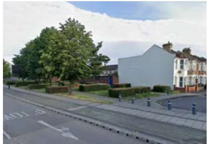
Developments along A13 incorporate a green buffer to protect surrounding homes, gardens and streets from poor air quality.
