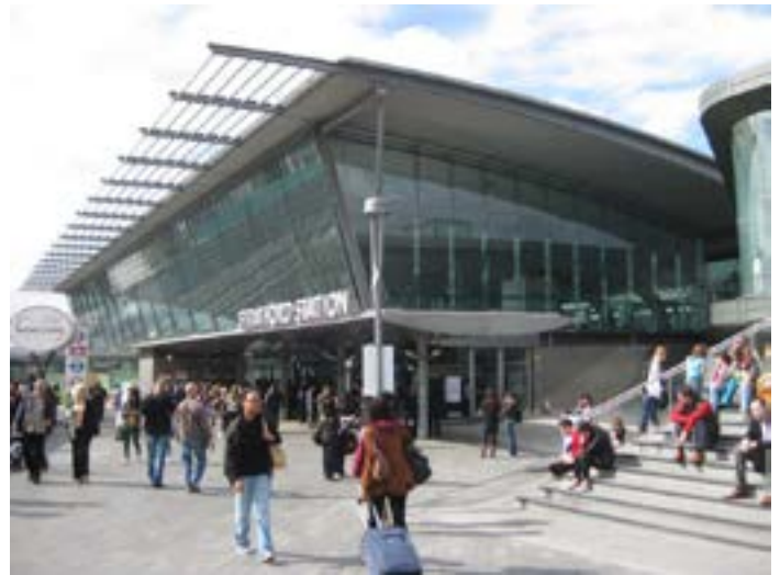
Places to wait and meet outside Stratford Station, Newham. A successful example of an arrival space provided outside key a public transport node that gives people sheltered, attractive places to meet, wait and sit.
