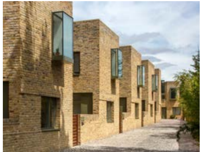
This mews street uses a stepped layout and massing in a backland site to maintain a sense of openness across the block. Oriel windows and frosted glass are used to animate the facade and reduce the visual bulk, whilst allowing in daylight without comprising privacy. Moray Mews, Finsbury Park by Peter Barber architects. Photo credit: Morley von Sternberg
