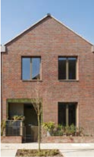
A terraced house with recessed porch, integrated storage, large ground floor window with deep reveals; and hard landscape boundary and defensible zone.
