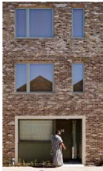
A terraced mews house on a semi-public street with ground floor kitchen, modest sized window, recessed porch and planting strip boundary treatment. Photo credit:
