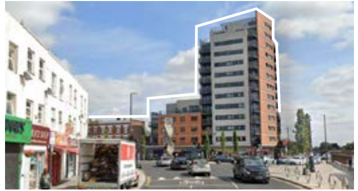
Image 1 - Maryland Station: Tall building integrated into a mid rise block, provides a scale transition with the low rise context while aiding wayfinding © Google maps
