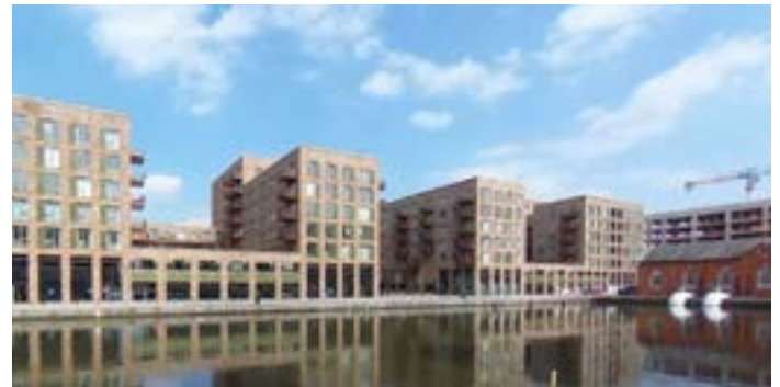
Image 3 - Royal Albert Wharf: Main building datum between 21m and 32m (ca. 7-10 storeys) without taller elements. © Google maps
