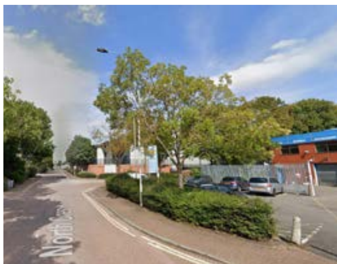
Typical shed landscape with some quality paving and planted trees and edges along the pavement.
