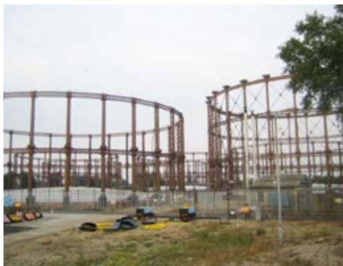
Grade II listed Bromley-by-Bow gasworks
