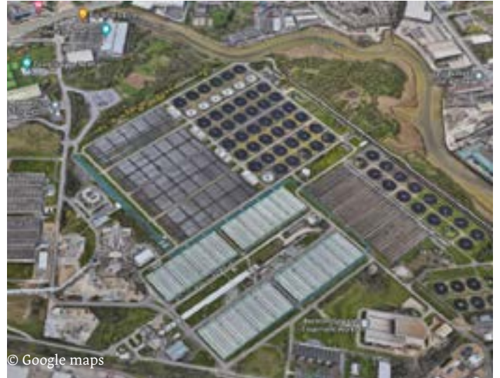
Beckton Sewerage Treatment Works.
