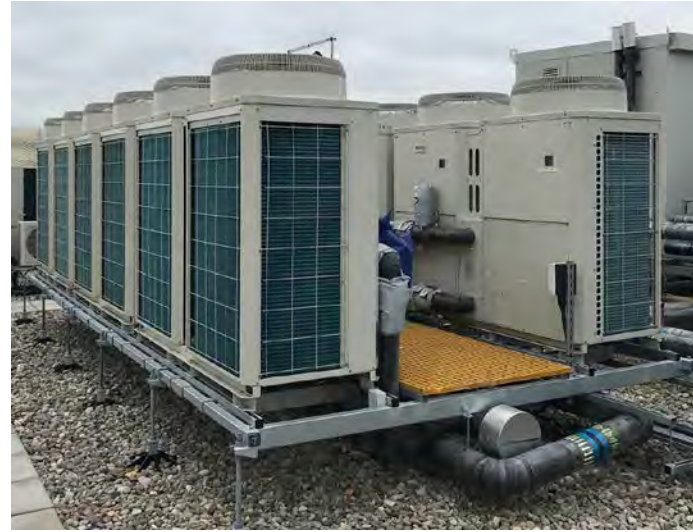
Commercial scale Air Source Heat Pump systems have been used for years in many types of non-domestic buildings (e.g. offices, hotels, etc.)
