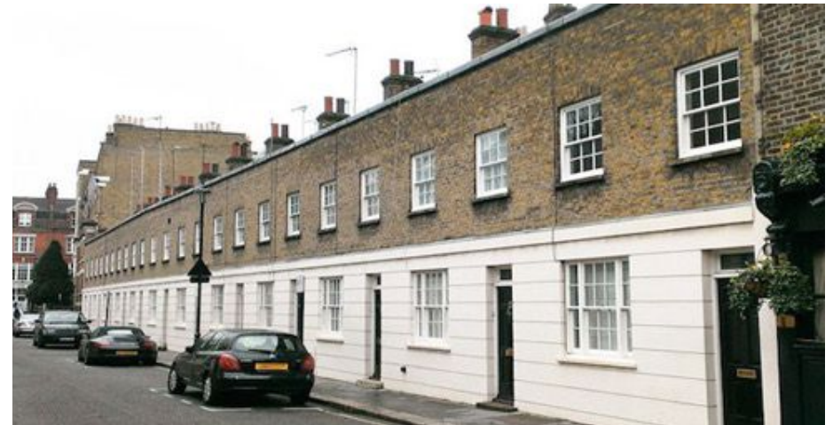
Two buildings in this row of London homes have been retrofitted to Passivhaus Enerphit standard, delivering around 75% better carbon savings over the neighbouring properties that were retrofitted to meet Building Regulations compliant standards (source: Passivhaus Trust)
