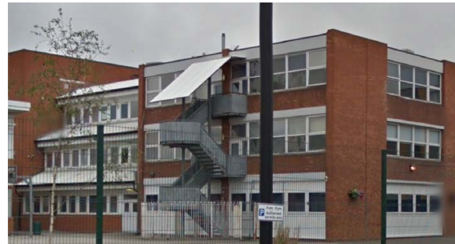
Forest Gate Community School, Newham – a mixture of buildings of different ages and construction, typical of secondary schools, with some new additions, some replacement windows and some new blocks
