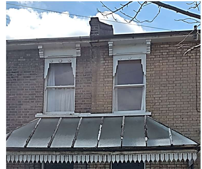
Traditional window blind box, rendered lintel and corbel 24
