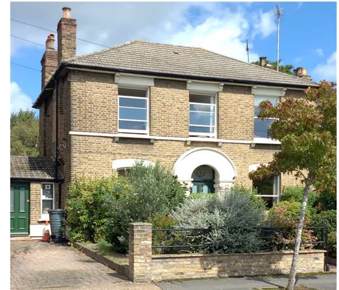
Double-hung sliding sash windows
