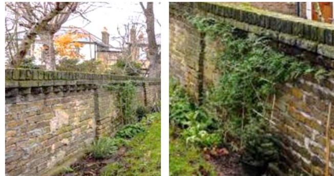
Traditional Woodgrange rear garden walls
