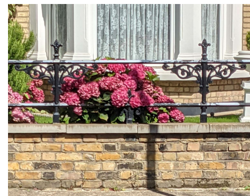
Woodgrange front boundary walls, gates and railings
