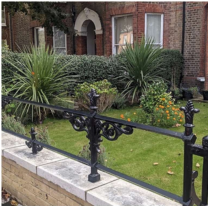
A green front garden with the Woodgrange style front boundary wall and railings preserves the street scene character.
