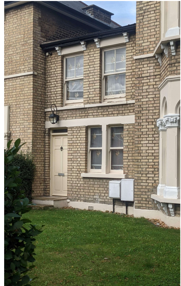
Original two storey annexe in Woodgrange
