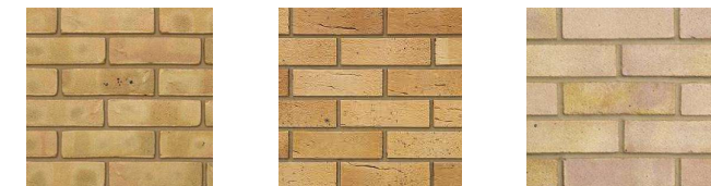
Bricks with an unacceptable appearance
