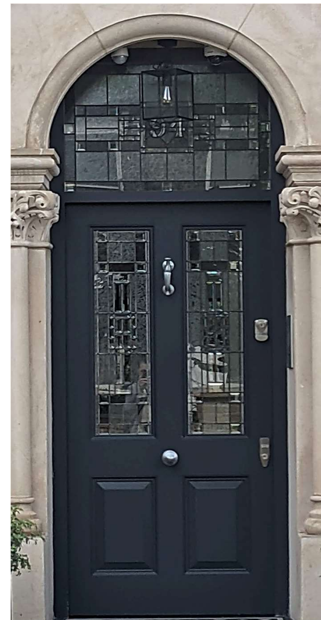
A new timber four panelled half-glazed door
