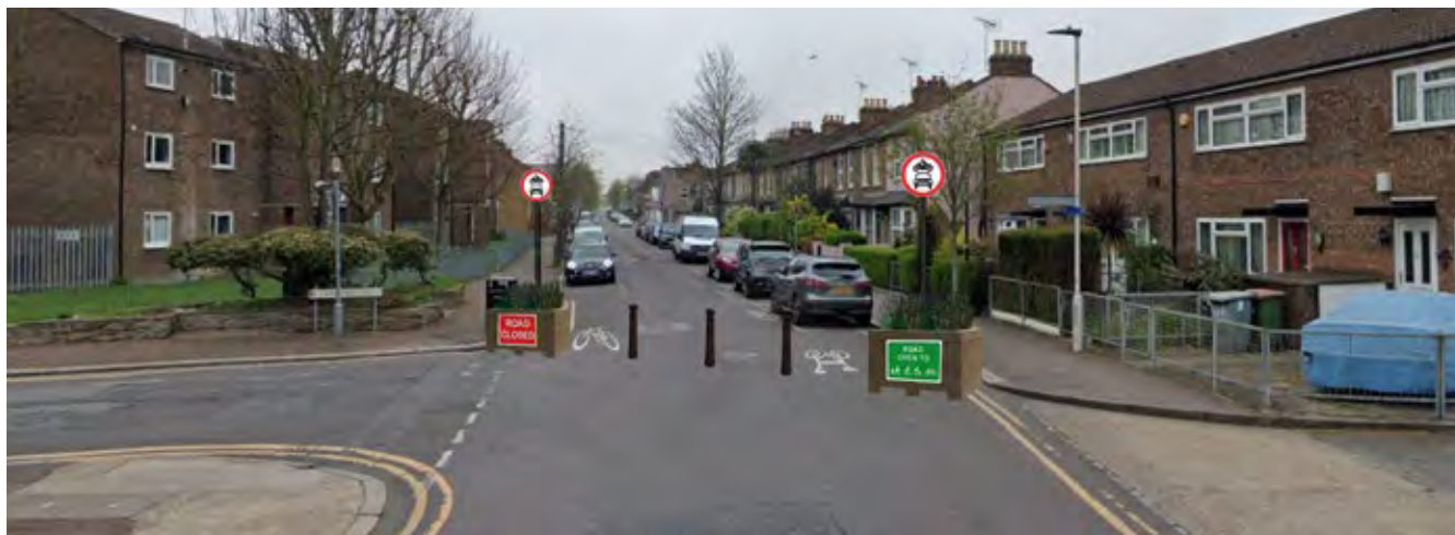
Indicative location of one of the modal filters on Odessa Rd, looking north towards Waltham Forest.
