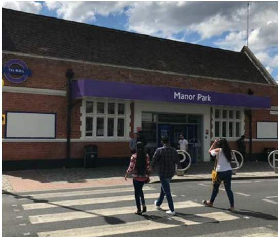
The station is located to the north of the local centre and at 30m of Manor Park open space.
