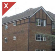
Figure 2.23c: Half-timbering has been wrapped around the side of the building but stops at the first window, highlighting that it is non-structural and is an accented detail.
