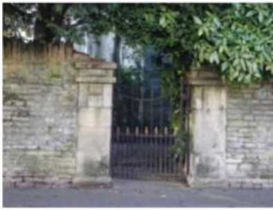
Figure 3.54: Pointed Cotswold stone wall with 'cock-and-hen' coping on Watermoor Road
