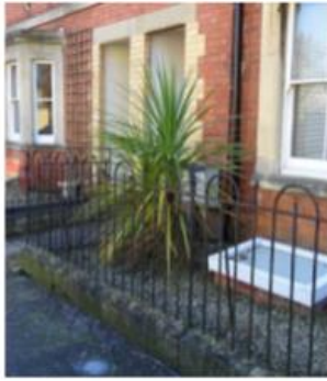
Figure 3.57: Metal Railings on top of a low stone wall on The Avenue
