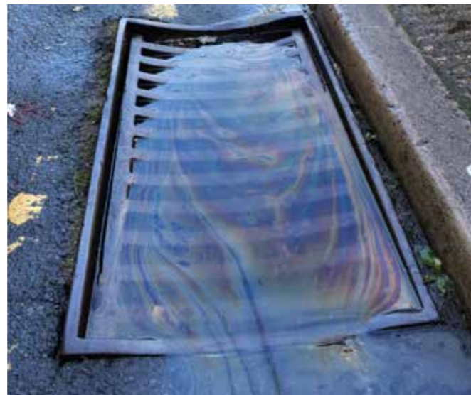
Pollution from roads and car parks is often visible - fuels, oil, heavy metals, tyre dust and silt all get washed into drainage systems.
