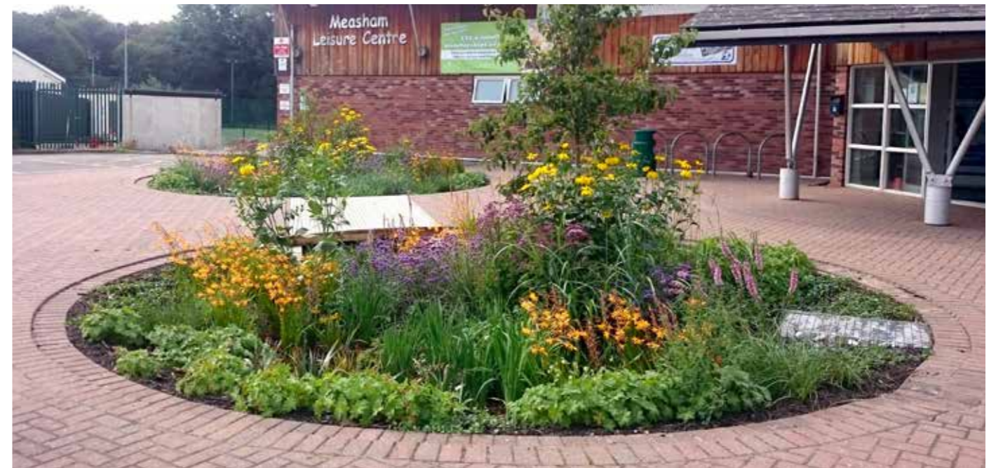
Two shallow raingardens provide storage at Measham Leisure Centre. Robust ground cover should persist through winter in order to protect soils.
