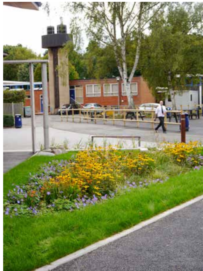
Longer SuDS grass as a filter strip between paved surfaces and a rain garden.
