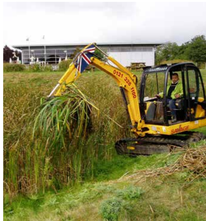
Hopwood Park MSA M42. A light tracked excavator removes aquatic vegetation to de-water next to the wetland, before moving to a wildlife pile.
