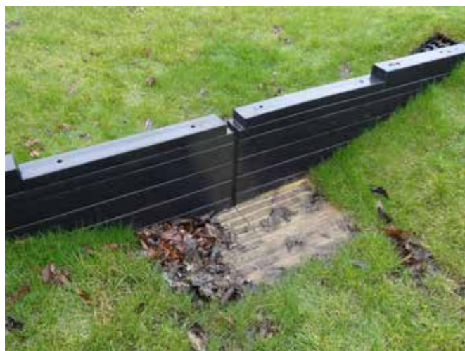
Flow controls in the landscape can make interesting features and help tell the story of how the system works. Although more prone to blockage, features such as this slot weir at Hollington School are very easy to unblock.
