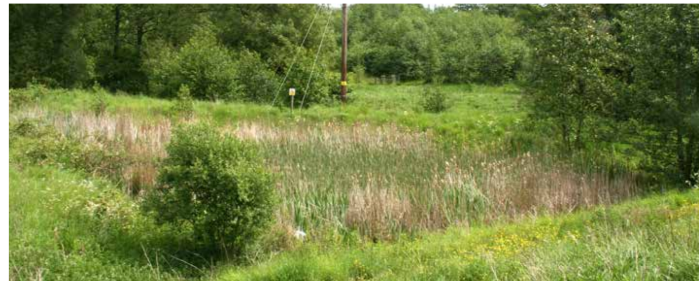
The final treatment stage at Hopwood Motorway Service Station. Monitoring has demonstrated that water of a very high quality (near drinking water standards) leaves site.
