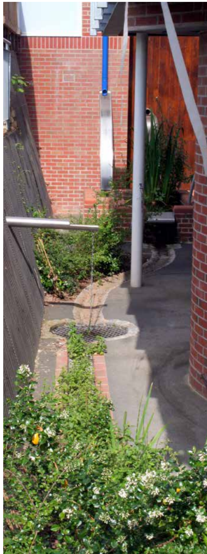
Fort Royal Primary School, Worcester. Mini-courtyard with rainchain, rain slide, raised pool and rill.
