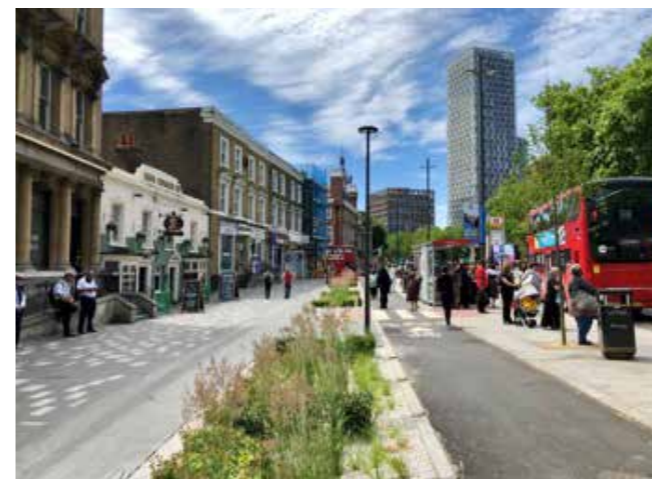
Fig.2 One of the 11 SuDS beds delivered by Newham across the Stratford Gyrotory
