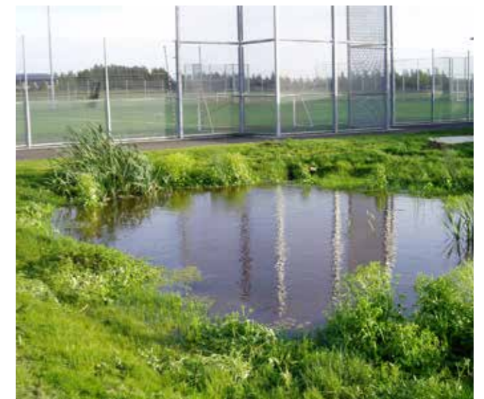
Pershore High School, Worcestershire. Swale conveyance into pond site control for final treatment and storage.
