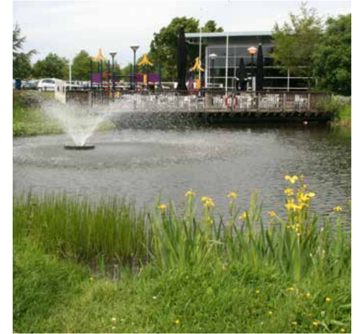
Hopwood Park MSA M42. Wooden terrace and balustrade with wet bench and planted aquatic bench protection to open water.
