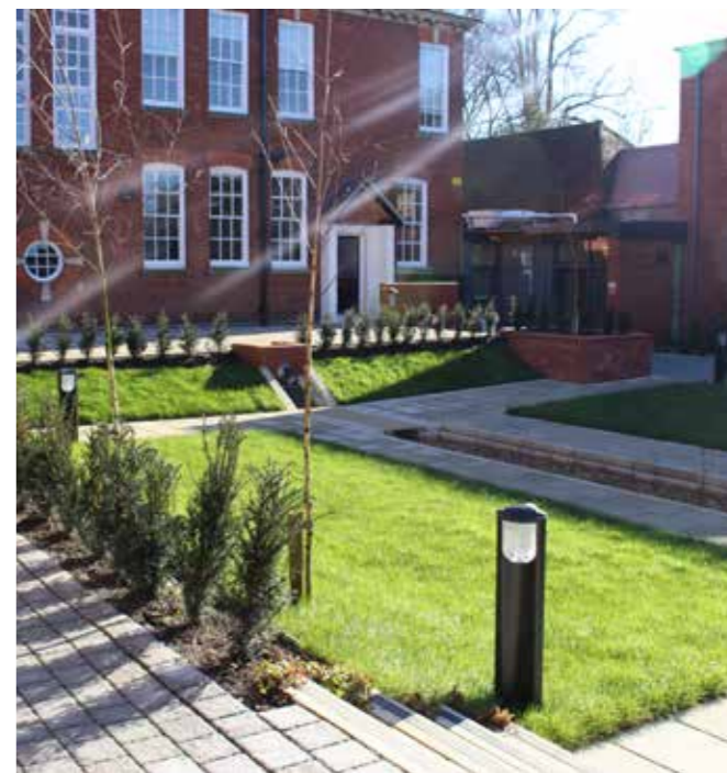
Parkside, Bromsgrove. Amenity grass shallow detention basin feature, integrated into site design, manages occasional extreme rainfall.
