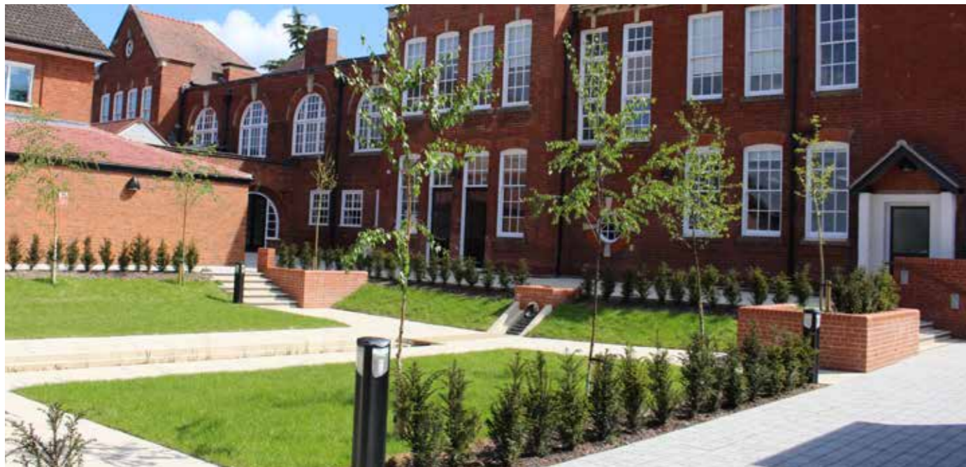
A sunken SuDS courtyard with solar water feature into a formal rill at Bromsgrove Civic Centre.
