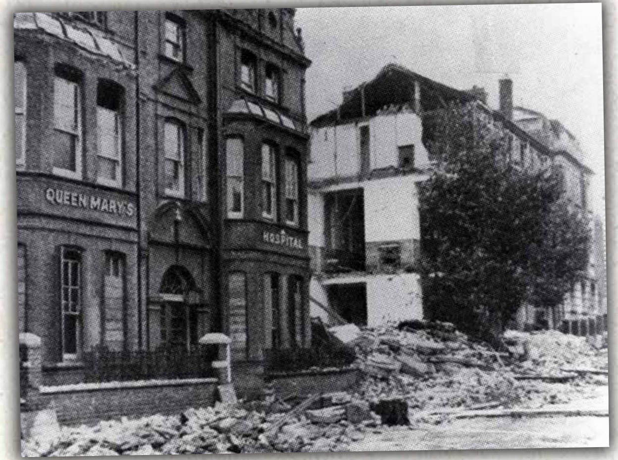
Queen Mary’s Hospital — 7 th September 1940 Two of the wards with staff quarters above were demolished by a direct hit from a high-explosive bomb at 6.10 p.m., killing six patients and two nurses. © London Borough of Newham
