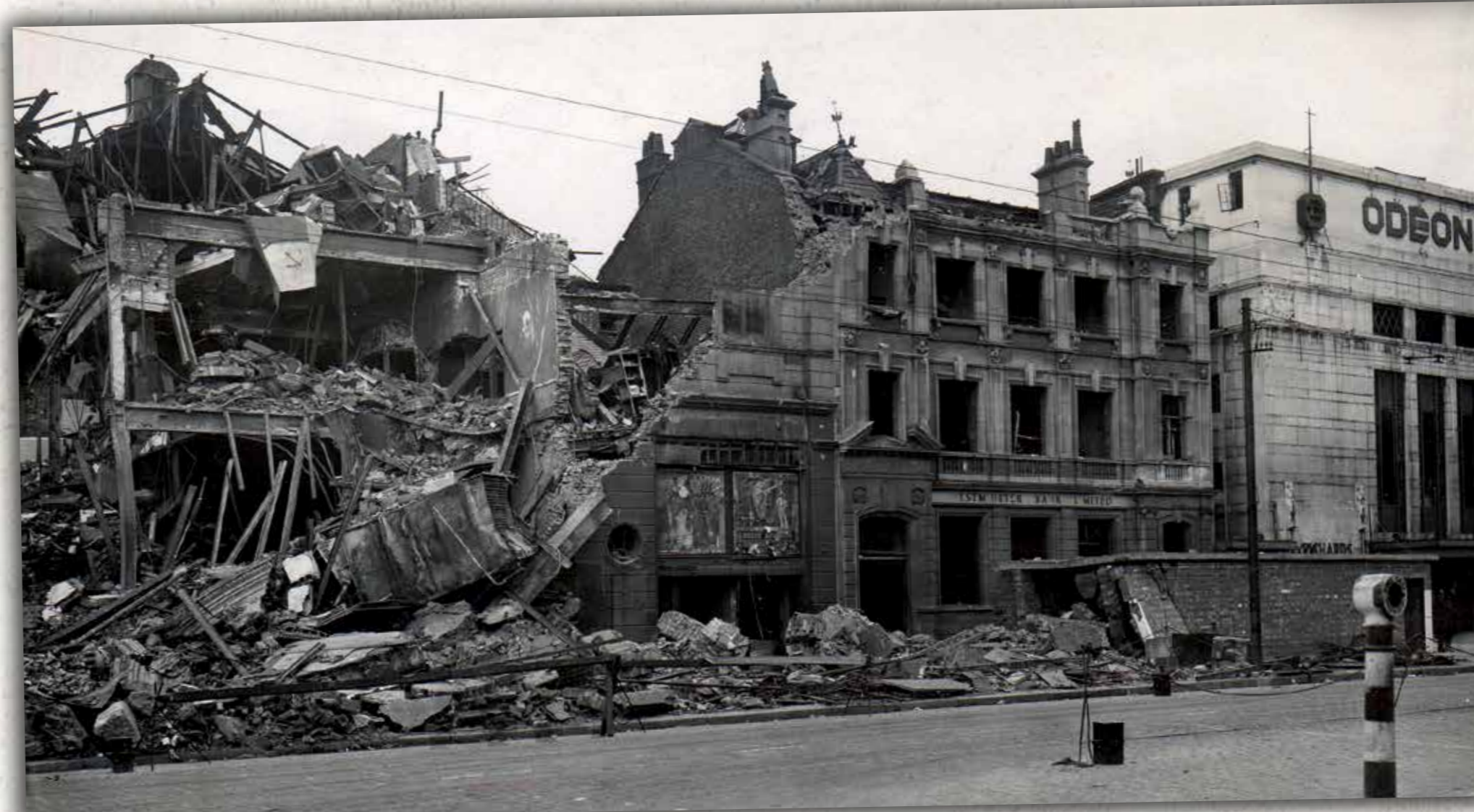
Romford Road, Forest Gate — 29 th April 1941 The Queen's Cinema was completely destroyed and blast damage can be seen on the adjoining Westminster Bank and the public air-raid shelter. © London Borough of Newham
