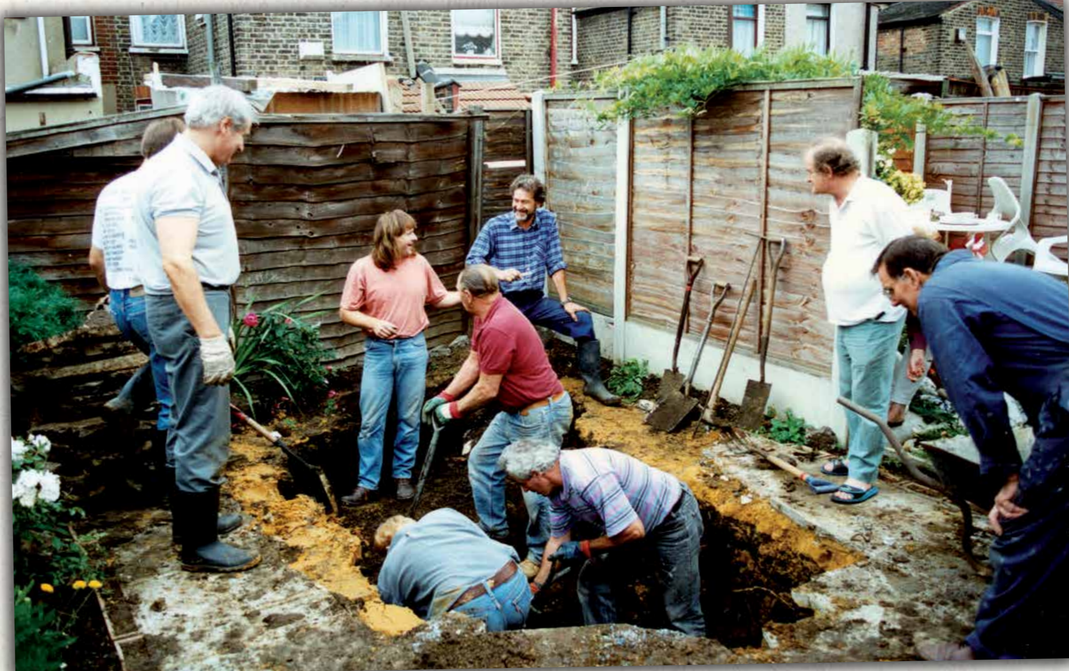
Excavation at Ranelagh Road, West Ham The After the Battle team at work in the rear garden of 75 Ranelagh Road in 1996. © Winston Ramsey
