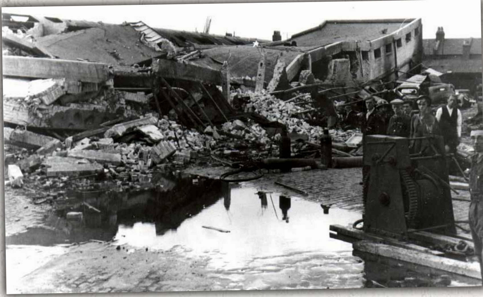
The ARP Depot and Ambulance Station, Abbey Road The depot took a direct hit on Black Saturday. Thirteen men were killed when a high-explosive bomb caused the building to collapse at 7.15 p.m. © London Borough of Newham
