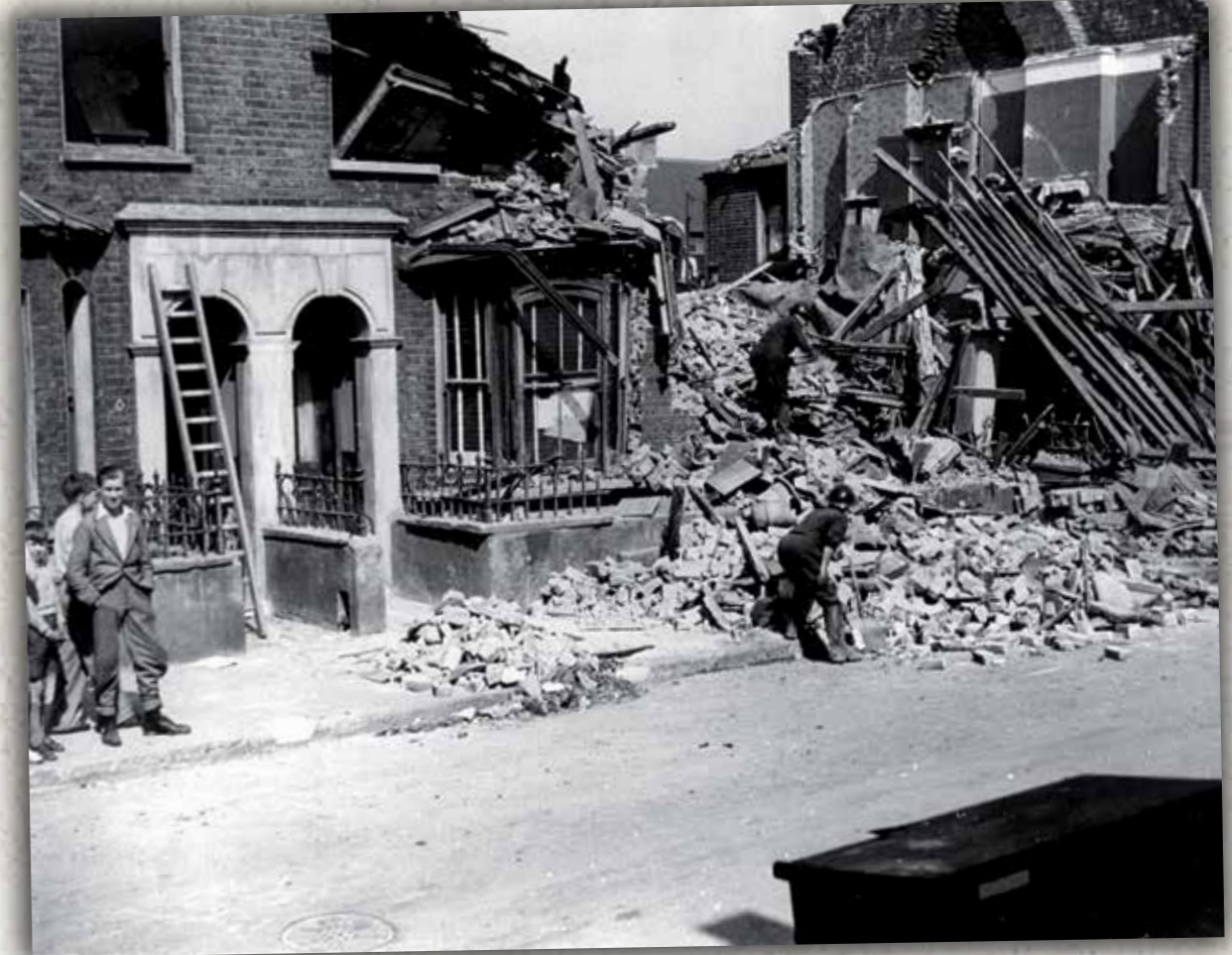
Cundy Road, Custom House — 6 th September 1940 Damage caused by a high-explosive bomb which fell at 9.43 p.m. © London Borough of Newham
