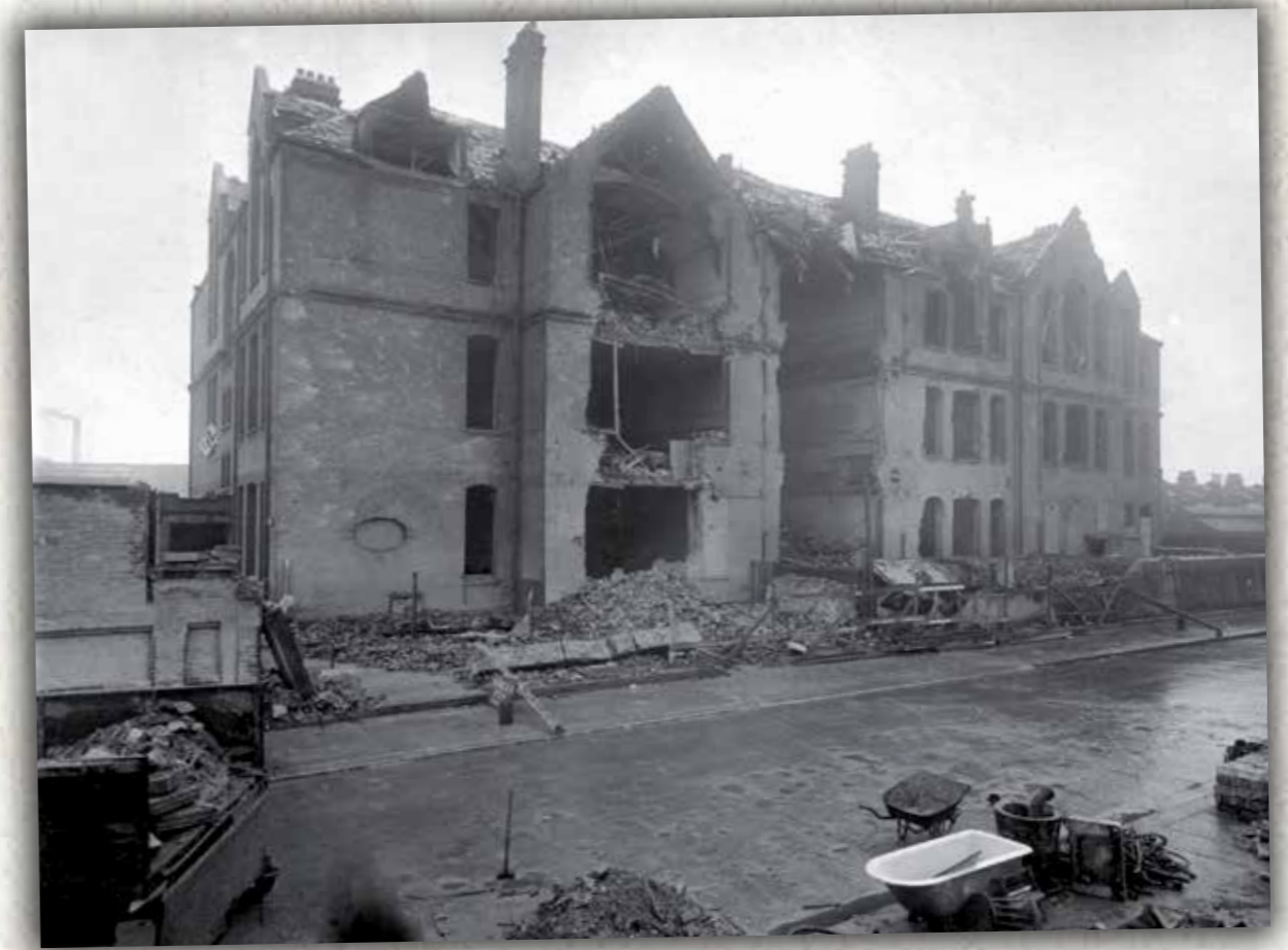
Frederick Road School, Canning Town (seen from Invicta Road) — 31 st March 1941 The school suffered four attacks between 7 th October 1940 and 19 th April 1941, being hit by incendiary, high explosive and delayed-action bombs. © London Borough of Newham
