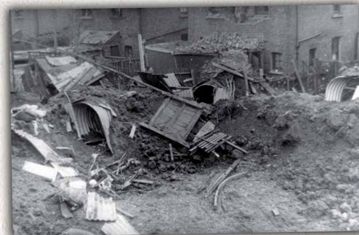
Anderson shelters in Croydon Road Plaistow These corrugated iron shelters, partly submerged and covered with earth, could withstand all but a direct hit. © London Borough of Newham
