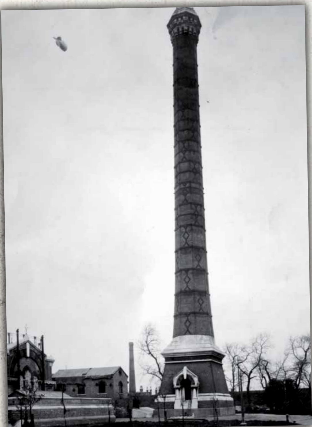
Barrage Balloon over Abbey Mills Pumping Station The war office decided that the risk of one or both of the 210 feet-tall chimneys being hit by German bombs was significant, and could cause the chimneys to topple onto the station. They were therefore taken down in early 1940. © Thames Water
