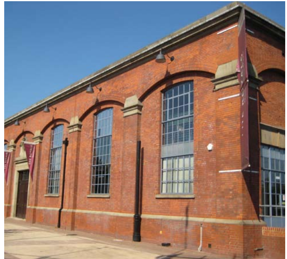
Compressor House, Royal Albert Dock
