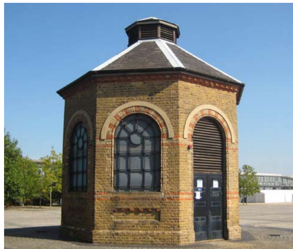
Connaught Pump House, Royal Albert Dock
