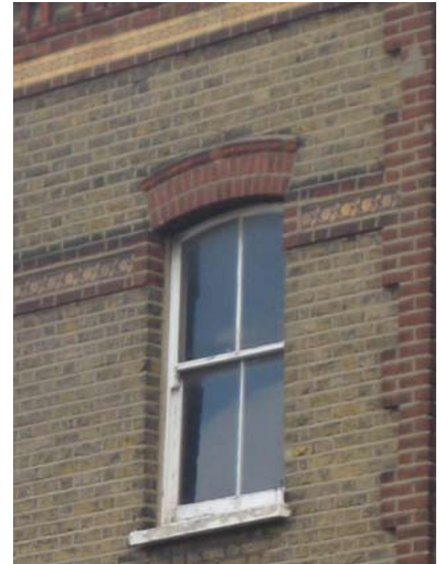
Tile detailing, 144 Barking Road, Canning Town
