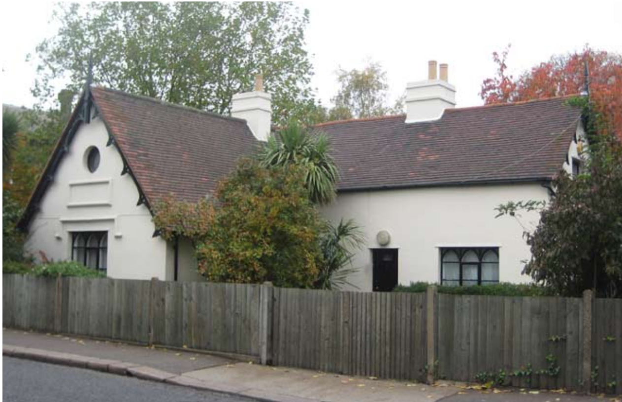
Tudor Revival Cottage, Portway, West Ham
