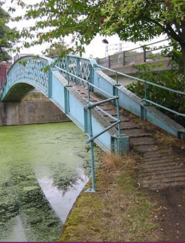
City Mill River Footbridge
