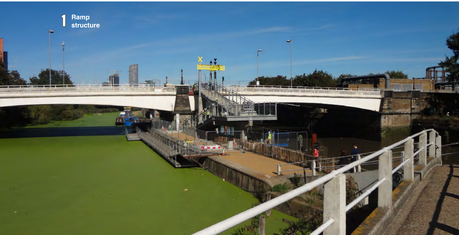
The new connecting ramp at Twelvetrees with its distinctive wayfinding structure
