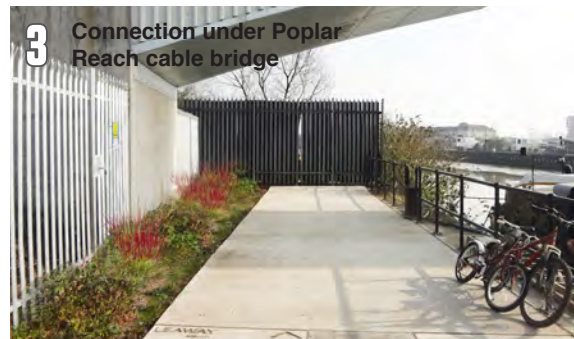
Access and landscaping have been delivered to enable a connection to Wharfside Road when the riverside along Crown, Mayer Parry and Whorlands Wharf is completed in Phase 2 of the Leaway.
